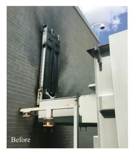
Upon receiving the call, the service team sprung into action to evaluate the situation, make it safe, and start preparing the switchboard for back-up power by disconnecting the damaged incoming bus-duct. Meanwhile, work began to source and deliver a large 1750KW, 600/347 emergency
